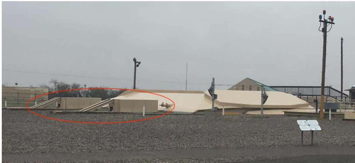
View of the closure door that rolls back to enable the missile to launch. The two huge concrete blocks in the red oval prevent the door from opening more than half way.
